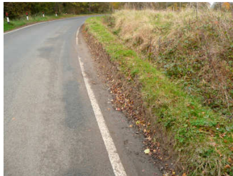
Example of verge erosion
