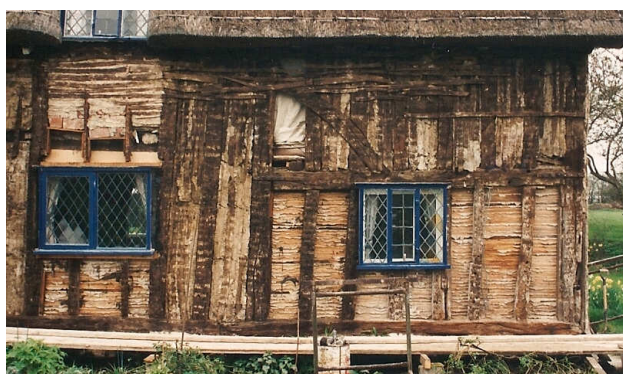
Timber framing under refurbishment
