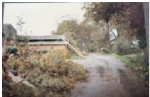
Storm damage, Green Street by Grange (now Griffin) Farm, October 1987.
