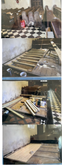
May 2016, St Mary's church, Great Canfield. A section of floor in the church was rotten and Charlie Barker repaired it. The photos show pews clustered together away from the work, joists in preparation and installed, and the repaired section with new floorboards in place.
