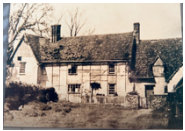
Another view of Ashfield.
