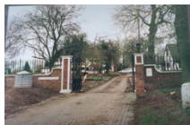
Old Barn House, Lower Road, January 2001, prior to demolition and development of Badgers.
